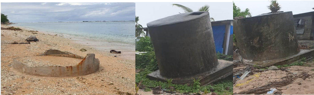
Figure 2: Fallen & broken concrete water tanks, Nanumea, 27 July 2020
